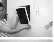
4 Align the speaker in position and tighten the screws evenly to secure the unit.
